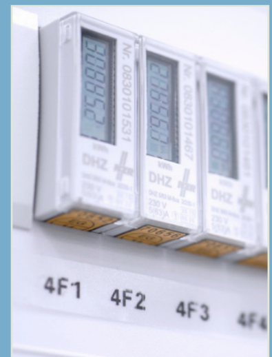
Certified electricity meters per customer and circuit for monitoring and billing purposes.
