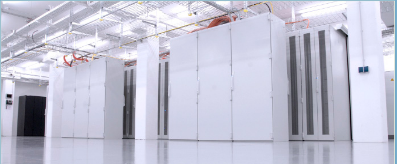
Ventilated customer racks (rear) with separate fiber and copper cable trays on top. Central MMR/ODF racks (front).
